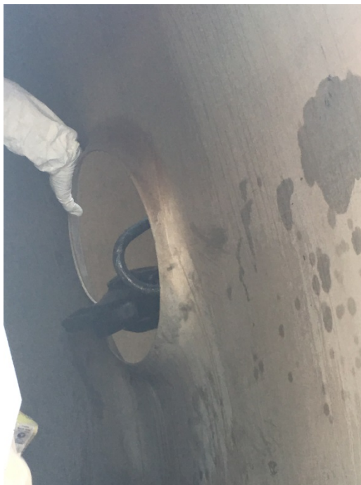
Access hole in baffle
